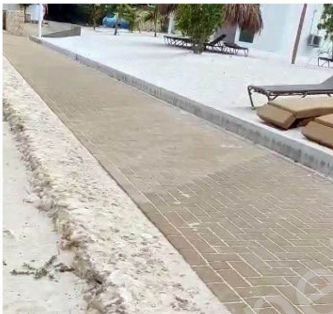
Figure 3. Footpath with retaining wall on the right side. Artificial beach sand is on the right side of the wall. Some natural sand is visible on the left of the picture.
